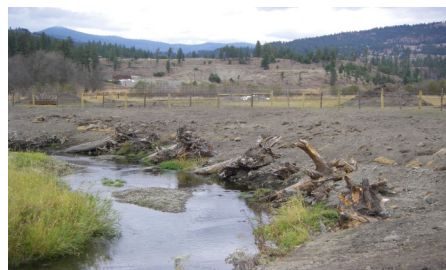
Top: Steep high banks are prone to crumbling in to the stream, unleashing tons of sediment. Bottom: Banks have been resloped and the toes protected with woody material. The banks and surrounding buffer will be revegetated. Protective fencing has been installed.
