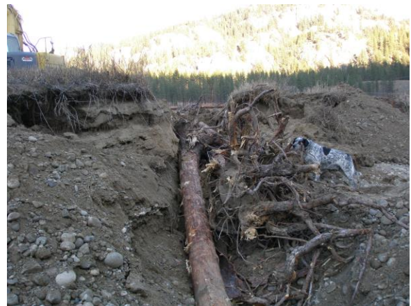
Large woody debris being buried in bank to stabilize it.
